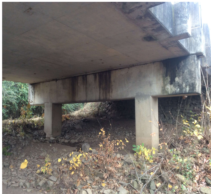
PHOTO 1 Description Intermediate bent caps have water stains that indicate deck joint leakage.
