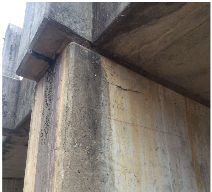
PHOTO 2 Description The Rt side of Bent 4 has a 12" delaminated area on the Span 4 side of cap.
