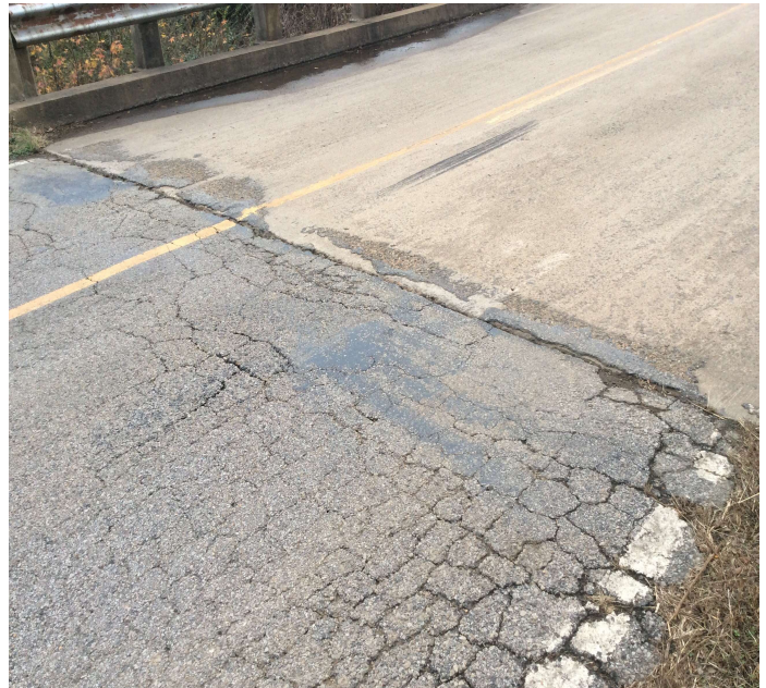
PHOTO 2 Description The approach roadways have minor asphalt settlement at the bridge ends. Bent 1 (West) bridge end pictured.
