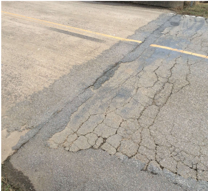
PHOTO 1 Description The approach roadways have minor asphalt settlement at the bridge ends. Bent 6 (East) bridge end pictured.
