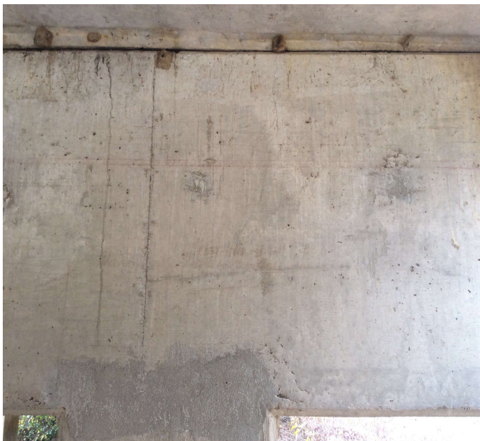
PHOTO 3 Description Intermediate bent caps have vertical hairline cracks over the exterior face of the columns.
