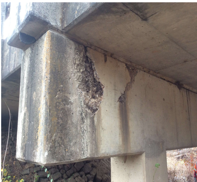
PHOTO 4 Description The Lt side of Bent 5 has a 36" delaminated area on the Span 4 side of cap.
